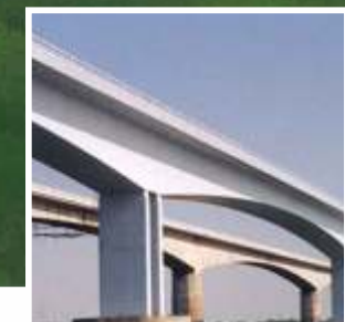
NAIGAON E/W BRIDGE
